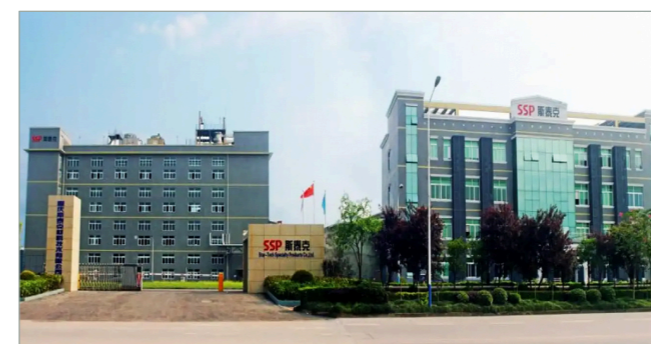
SSP Headquarters in Chongqing, China
