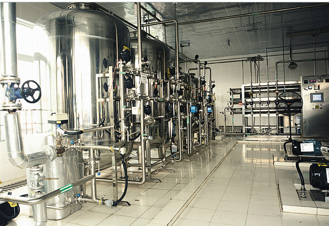
SSP Production Site, Chongqing, China
